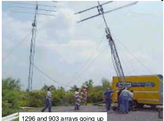
1296 and 903 arrays going up
